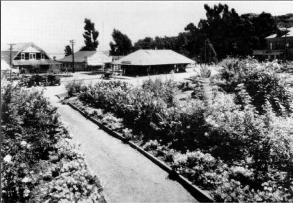
Figure 2.2.2.a. Cortes Madera Village Square and Railroad Park, 1926.
