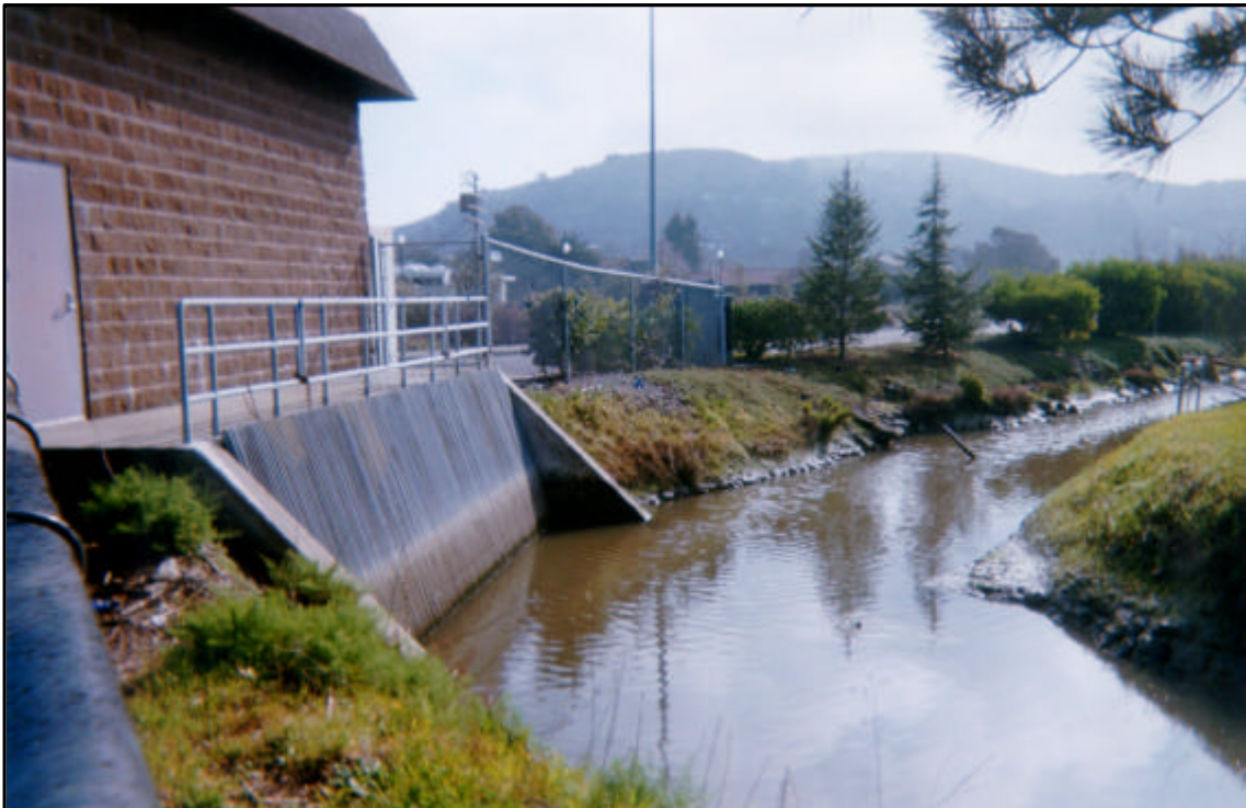
Pump Station at San Clemente Creek.
