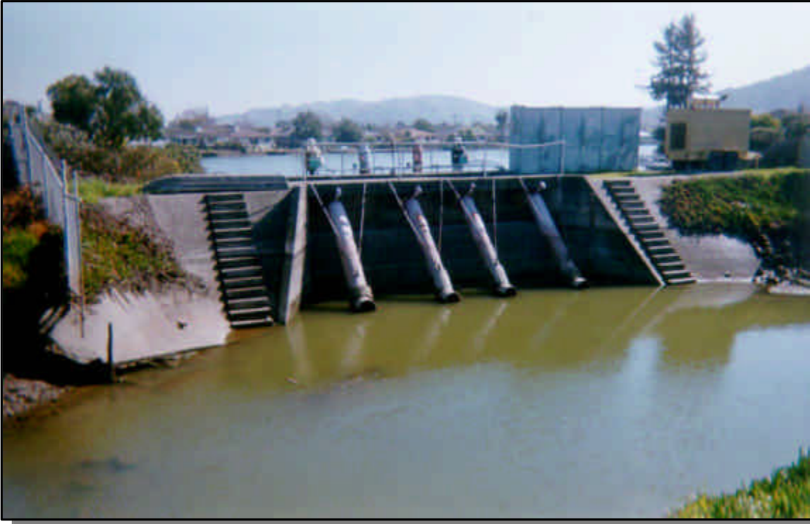
Pump Station at Lagoon No. 1.
